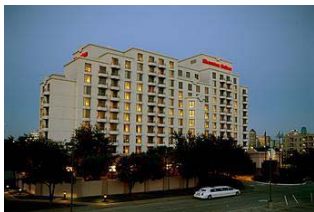
Sheraton Suites Market Center Dallas, Texas
